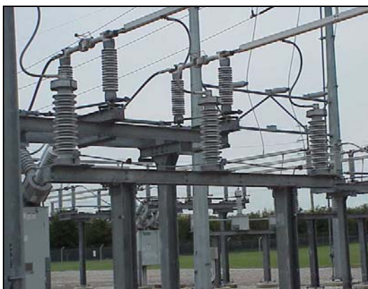
Figure 1. Failure of a 69 kV lightning arrester. This problem could have affected reliability of this power system by causing an outage to several thousands of consumers being served by this substation.
