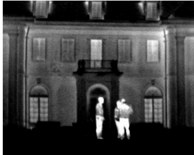
Figure 3. Oldfields Estate, front (east) elevation. The black and white thermograph (right) shows heat loss through windows and dormers. The human figures appear warmer than the building.
