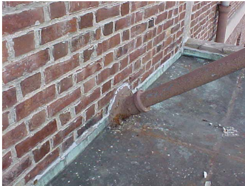
Figure 3. Location 2, Building K, east elevation.
